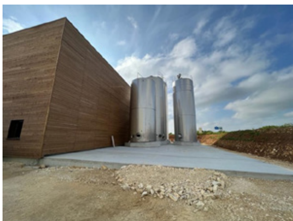
A building has been constructed to house the prototypes and the ZEUS laboratory. ©OiEau
